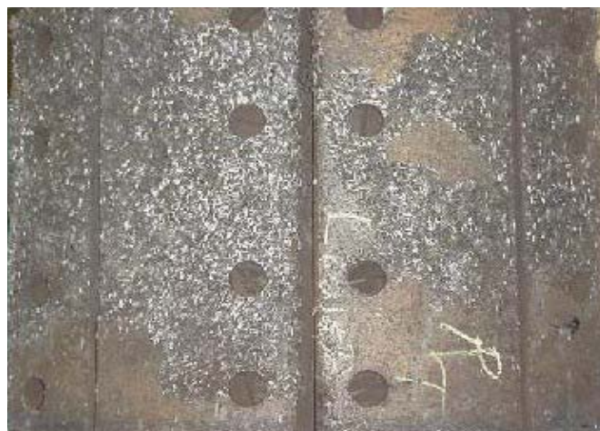
Figure 2. This photo shows damages to the lining surface from lining-to-drum bonding
