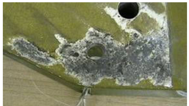
Figure 26 – Example of Corrosion on Stub Wing and Wing Attachment Fittings (Cessna 402C)
