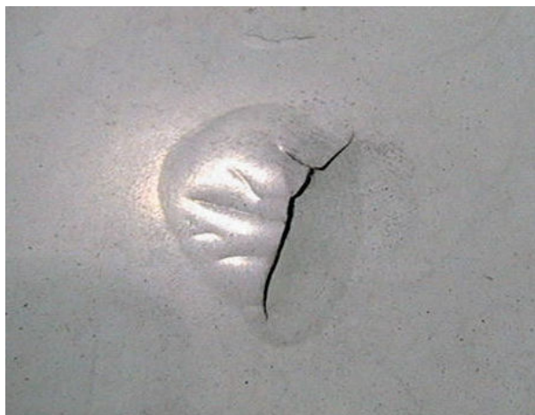
Figure 6 – Paint Bubble in Skin that Cracked Paint
