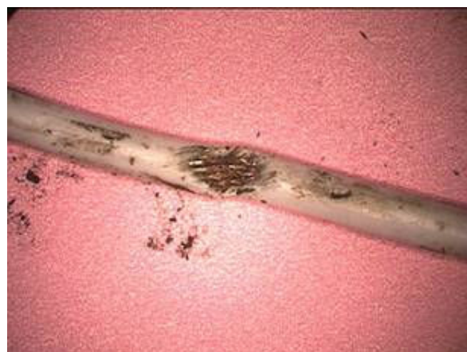
Figure 13 – Example of Exposed Inner Conductor
