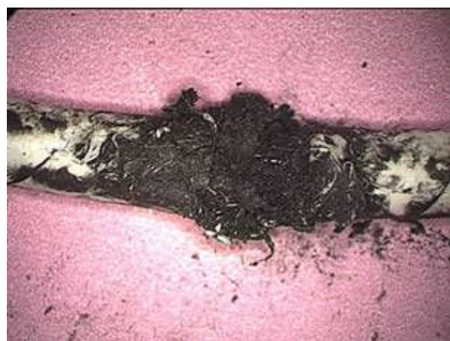
Figure 14 – Example of Heat Damage
