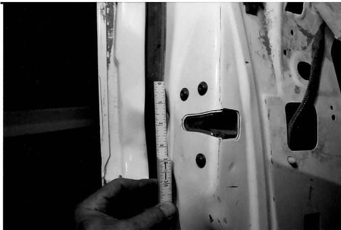
Figure 3. Latch was functional but with a slight expansion of the fishmouth. Ruler indicates ripples in end panel from vertical loads.
