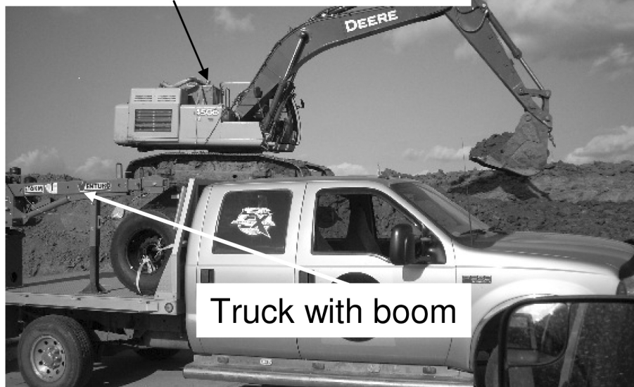
Figure 2. Truck with boom used to install PEMS units on the construction equipment. In the background is an excavator with a PEMS unit installed.
