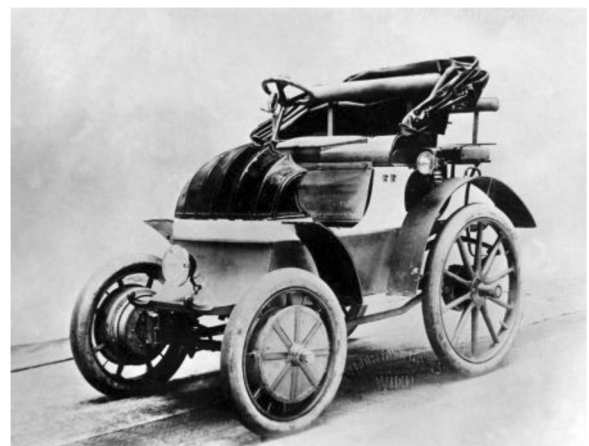
Figure 1. An early 1900s ‘System Lohner-Porsche’, propelled by in-wheel motors ( reference 2 )
