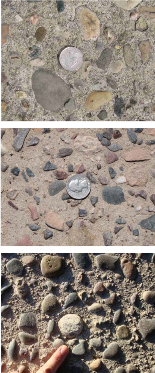
Figure 2. Photographs of coarse road pavements at Track 1 (top), Track 2 (middle), and Track 3 (bottom)
