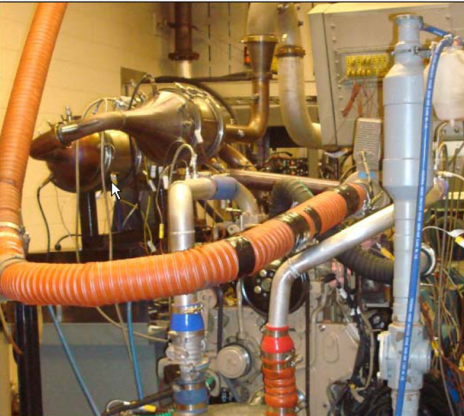
Figure 2. Engine and Aftertreatment System in a Test Cell
