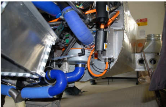
Figure 5. First and second stage compressor.
