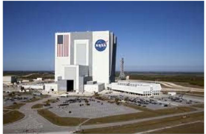
Figure 2. The Vehicle Assembly Building at KSC. Photo credit: NASA
