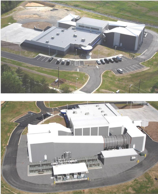
Figure 1. Aerial views of the Windshear Facility
