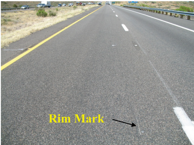
Figure 4. Rim Contact from Right Rear Rim
