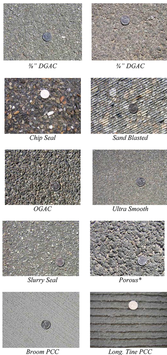
Figure 2. Test pavements at the Hyundai Kia Proving Ground (*Note: "Porous" is not actually porous)
