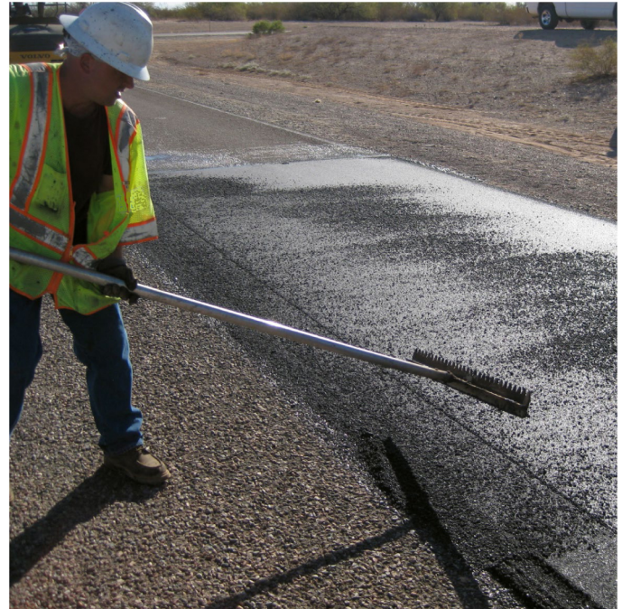
Figure 6. Using a lute to broadcast loose asphalt material across the mat is can lead to inconsistent and undesirable texture.
