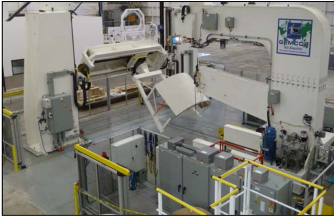
Figure 2.0. Installed CNC Composite Fastening System
