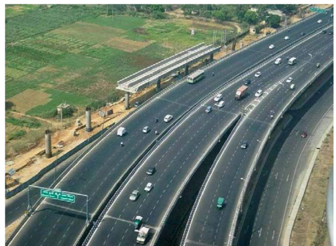
Figure 1. A dual carriageway section of National Highway 8 connecting Delhi to Gurgaon.
