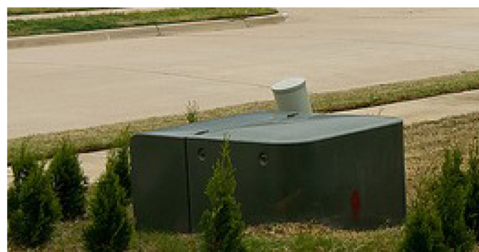
Figure 6. Pad-mount transformer
