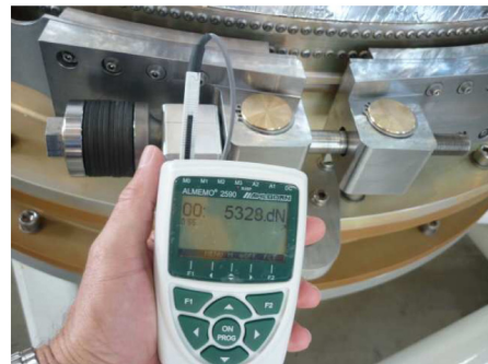
Figure 2. Tensioning process (use of load cells)
