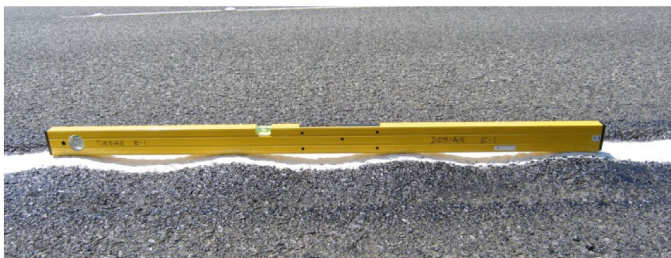
Figure 1. Photograph of the sinusoidal rumble strip profile as built
