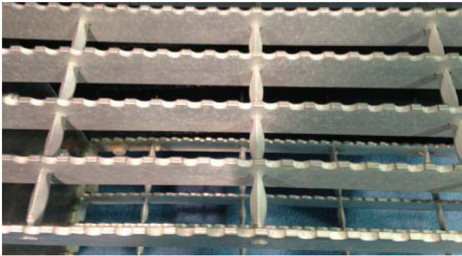
Figure 6. Example of machined step design.
