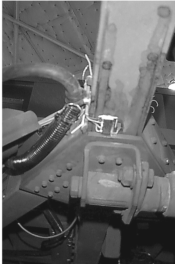
FIGURE 2 - LOCATION AND INSTALLATION OF THE STRAIN GAUGE ROSETTES
