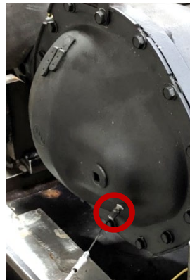
Figure 2 - Thermocouple for UUT temperature measurement
