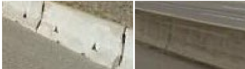
Figure 2 - New built (left, cluster 1) and old concrete divider (right, cluster 2)
