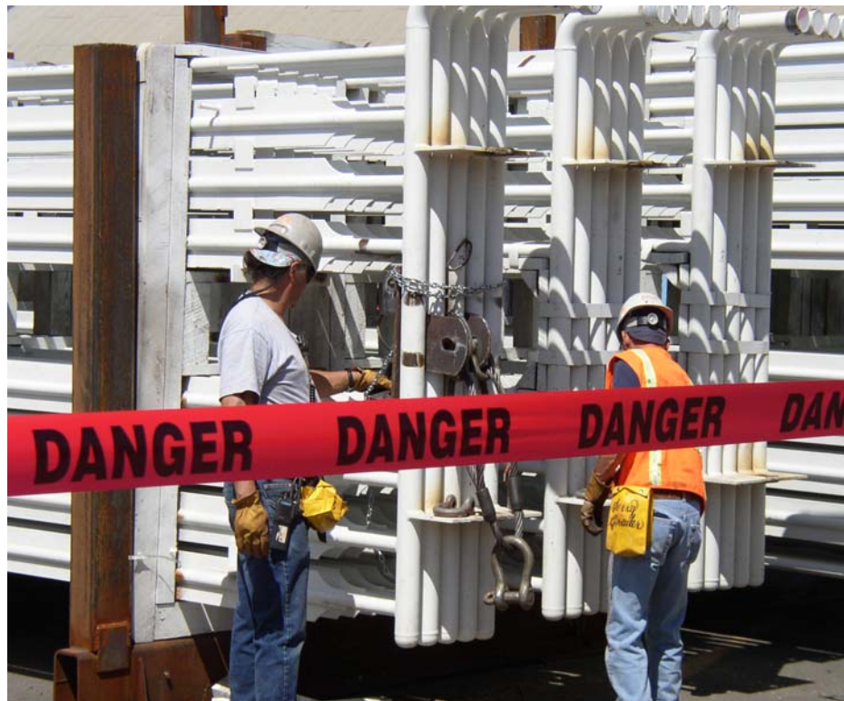
Fig. 1. Mini-header sheets pre-assembled for shipment in groups of five with upper headers vertical.
