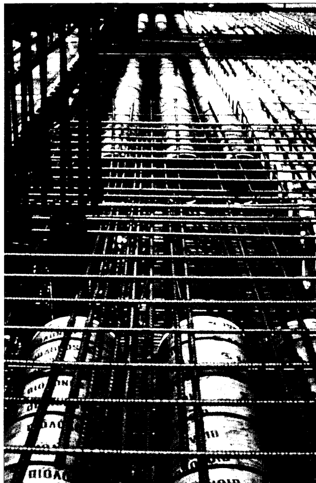
Fig. 5.5 — Voids are formed in the slab by laminated fiber tubes. The tubes are tied down with wire to prevent movement during concreting. (Photo courtesy of Sonoco Products Co.)
