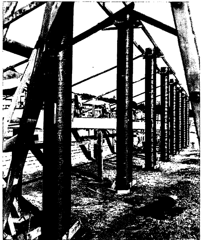
Fig. 5.7 — Fiber tube column forms require bracing to keep them plumb and a template at the base for accurate positioning.
