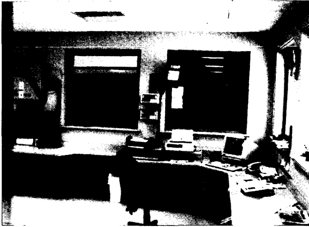
Fig. 2.9 — A batch plant control room where the operator can monitor the batch weights of materials, including admixtures. (Photo courtesy of Automated Control Technologies, Inc., and Stephens Manufacturing Co.)
