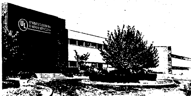
Melville, N.Y. Testing Station
