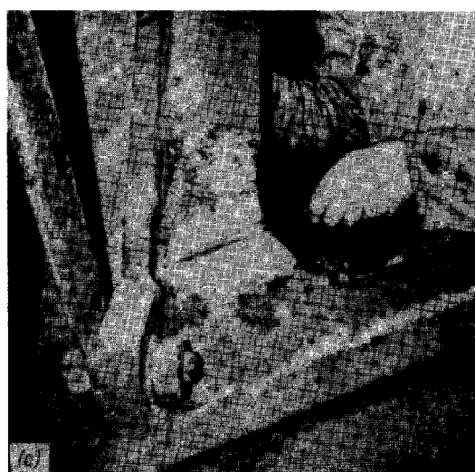
2 Osney Bridge showing: (a) cracks, dye penetrant tested, (b) cutting with hacksaw, and (c) nickel strip in place
