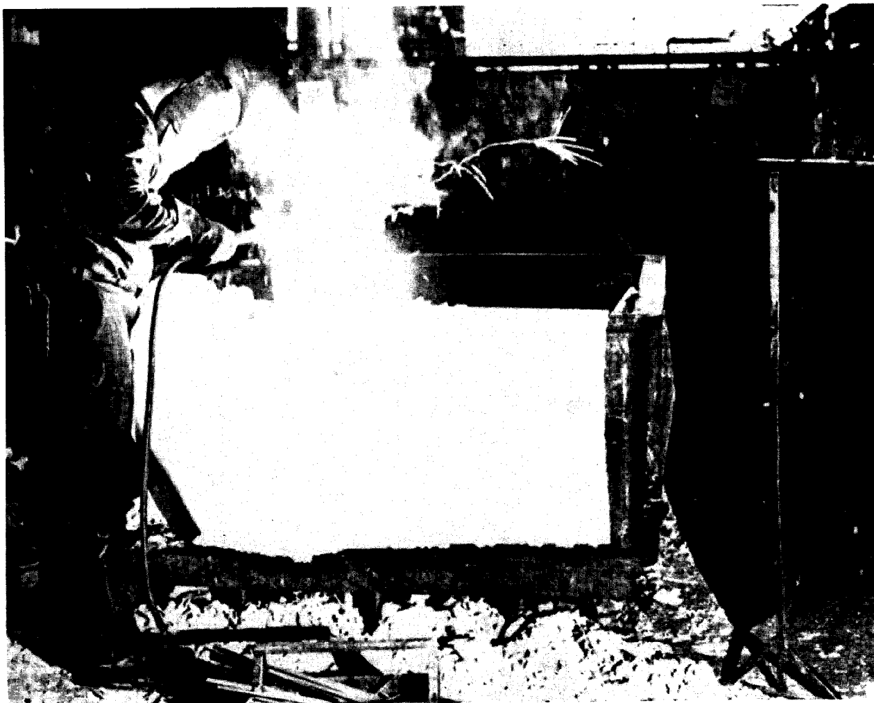
"Hot Arc" welding in progress on a gray cast iron casting
