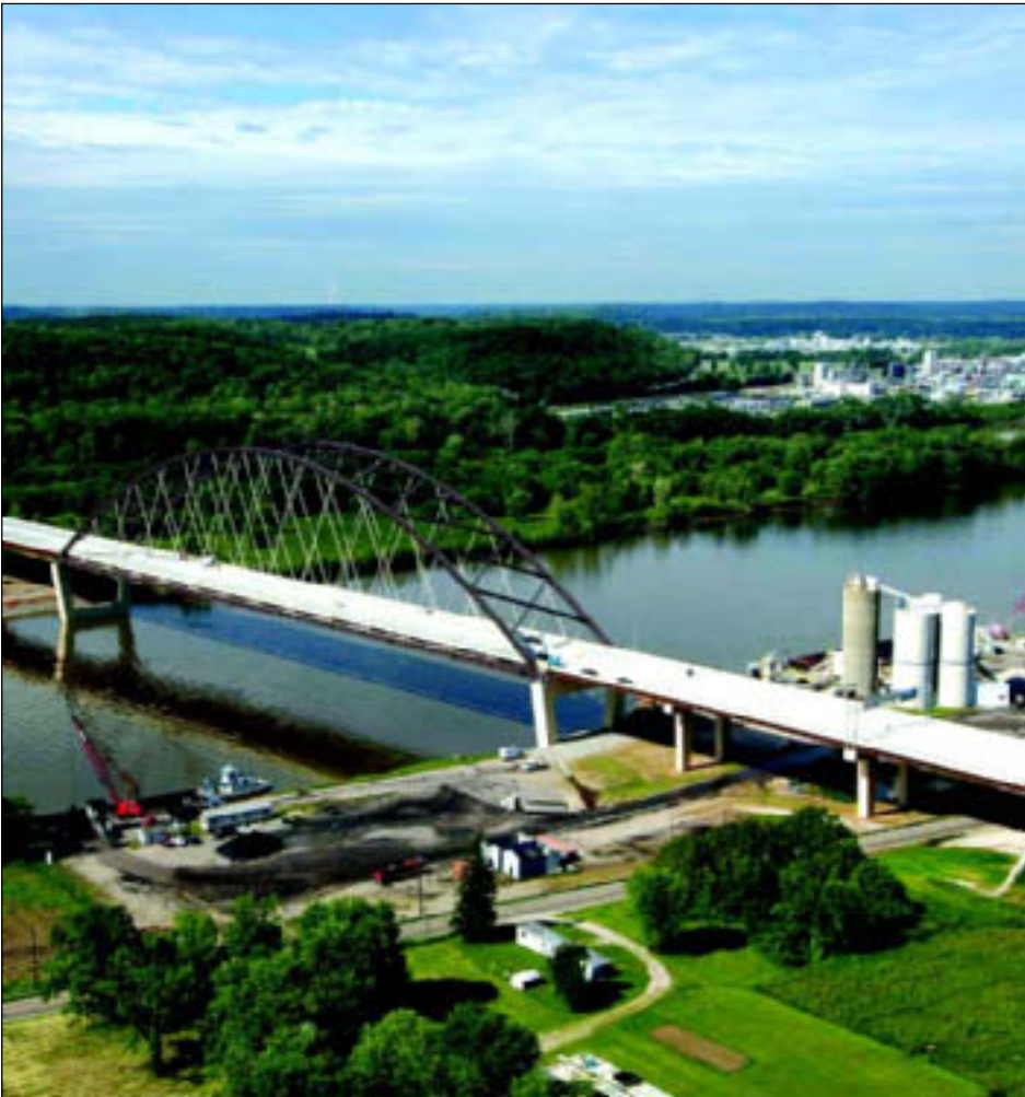
Photograph courtesy of W. Virginia Dept. of Transportation—High-Performance Steel Bridge over the Ohio River
